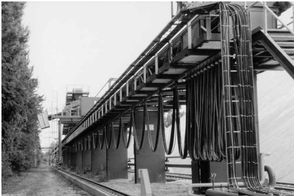
Vahle Flat Cable Festooning System for Stacker/Reclaimer Electrification
